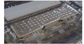
216,752 SF Class B Industrial Warehouse
